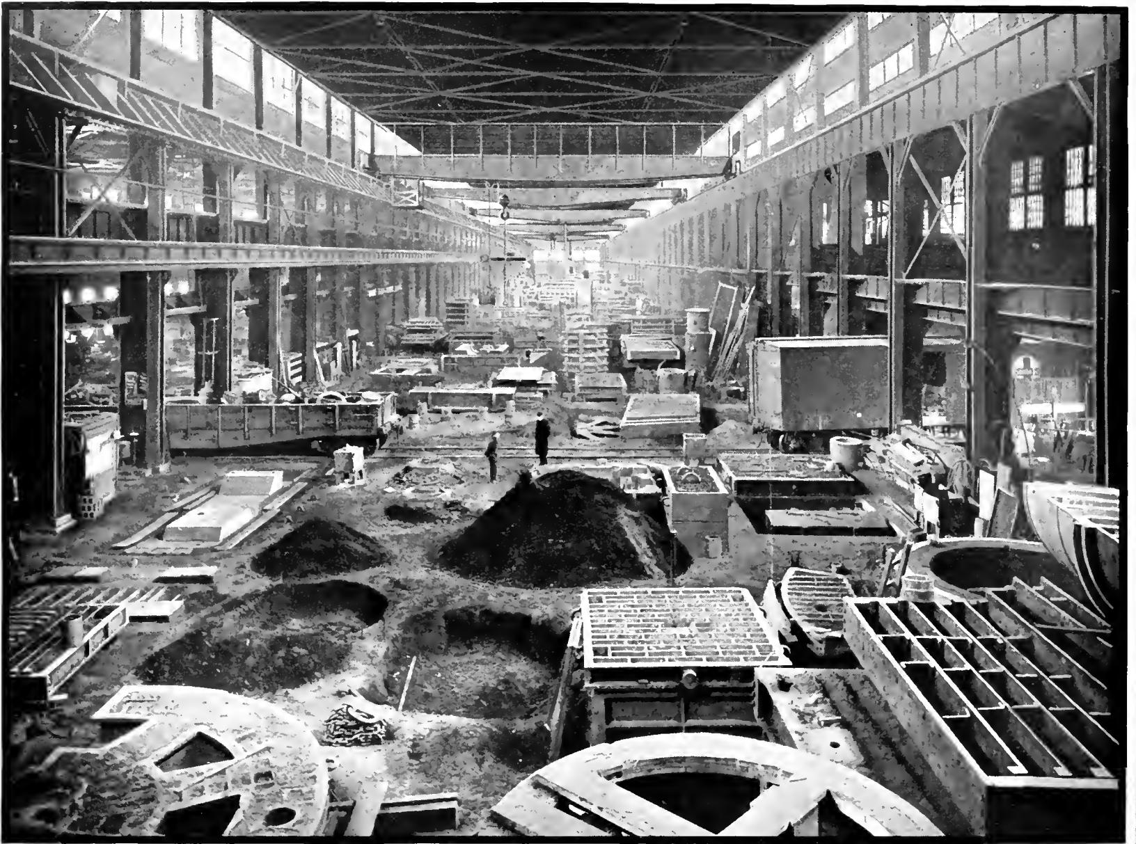
View of Main Aisle in Foundry Department
